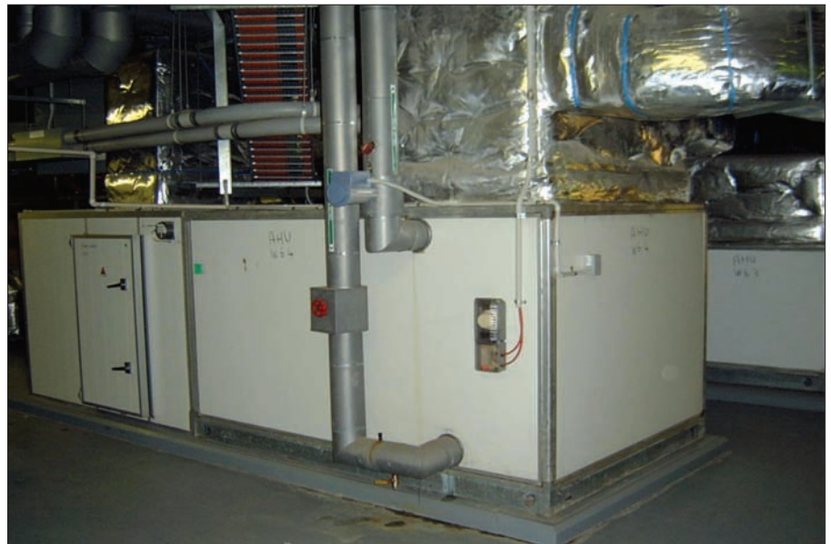
The existing building management system was reconfigured and reprogrammed.
